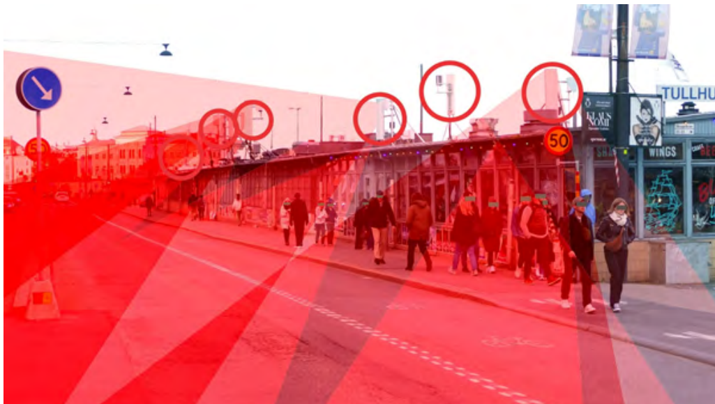
Figure 4: Low positioned base stations at Skeppsbron, Old City, Stockholm, Sweden
